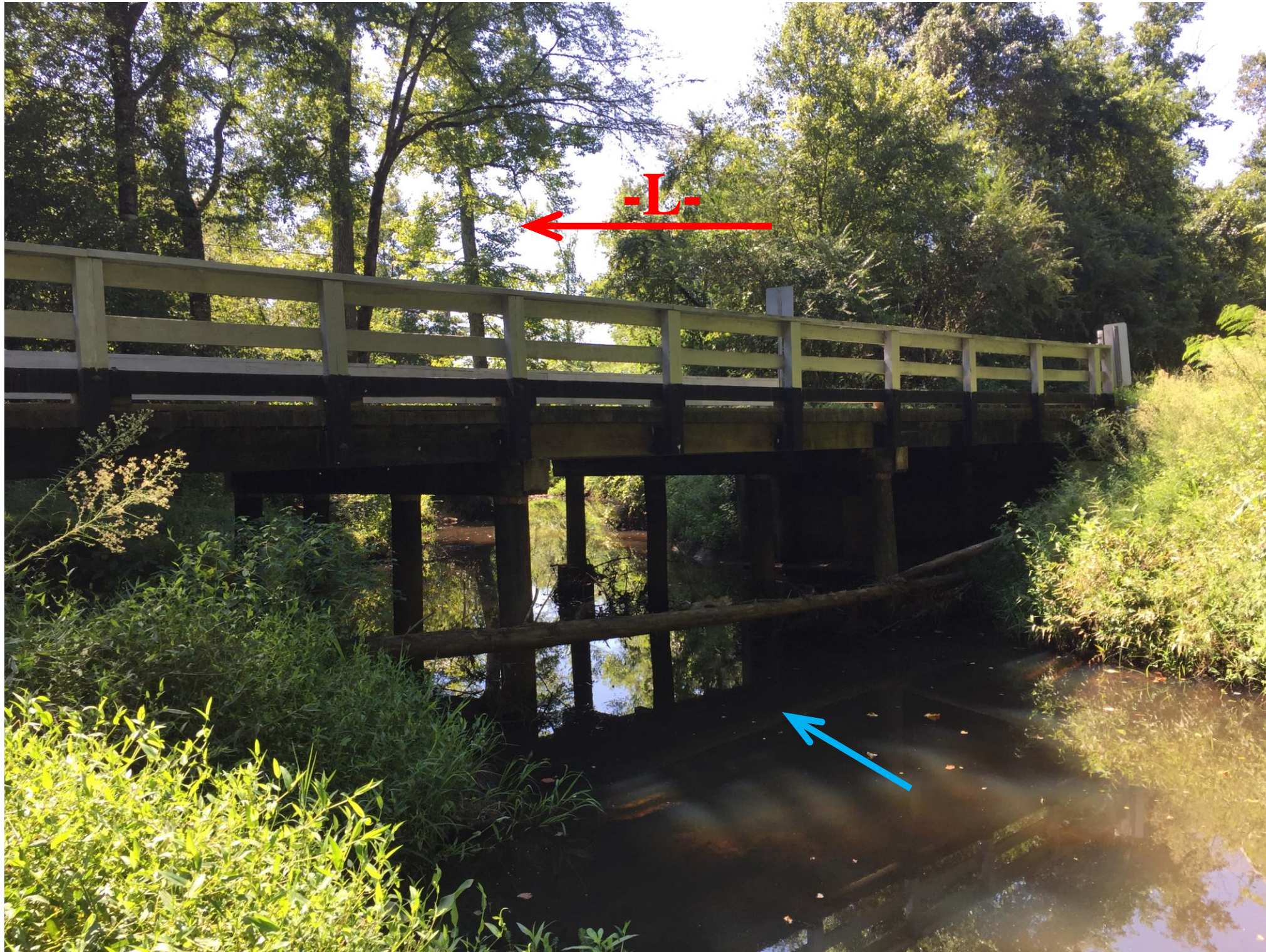
Looking South towards End Bent 1
